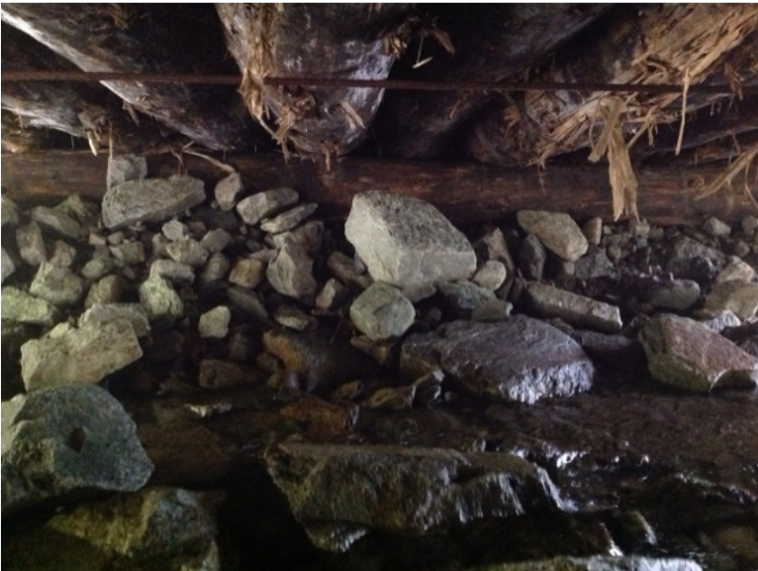
Left Bank Abutment when facing downstream
