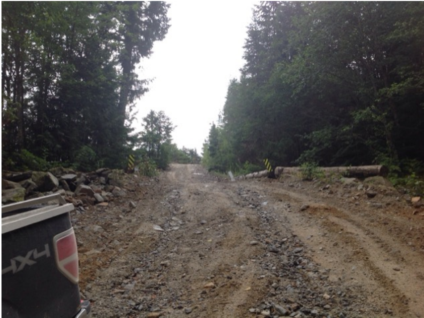
Approach from Left Bank when facing downstream - 26%
