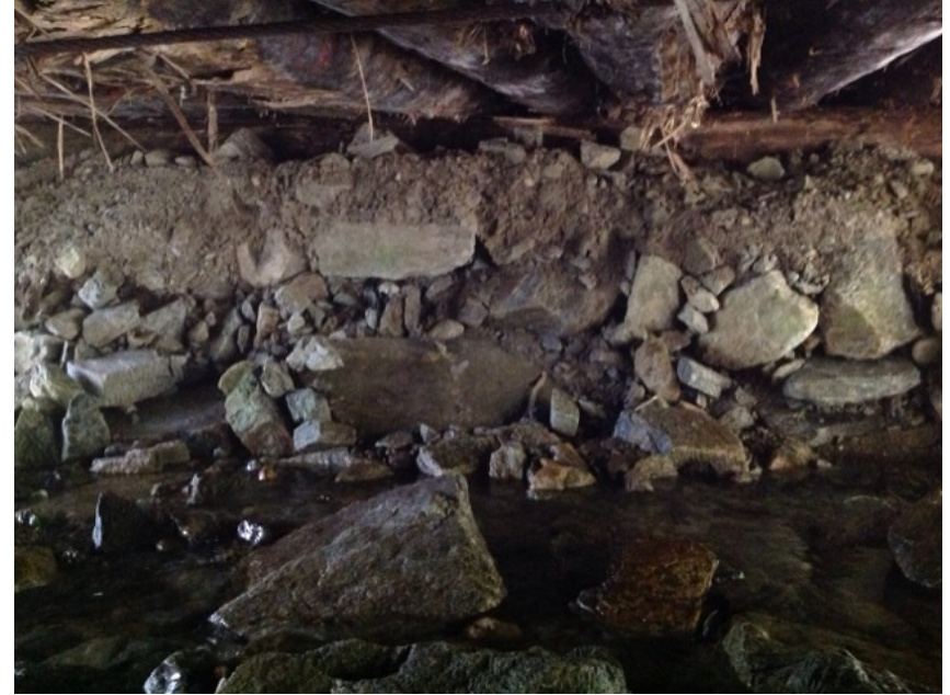
Right Bank Abutment when facing downstream
