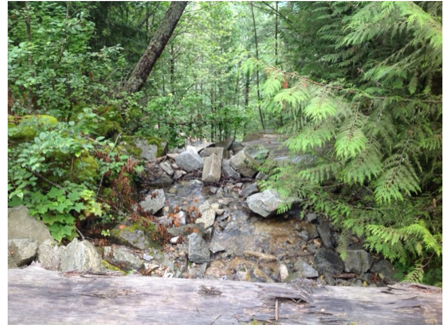
looking downstream from deck
